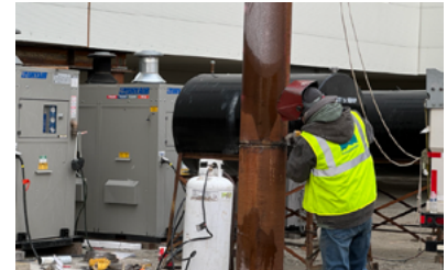
Splice welding of piles
