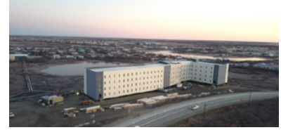
Exterior metal siding 90% complete
