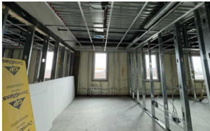
Staging sheetrock (post inspection)
