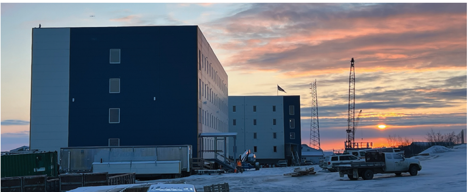
Staff Housing exterior view to the east
