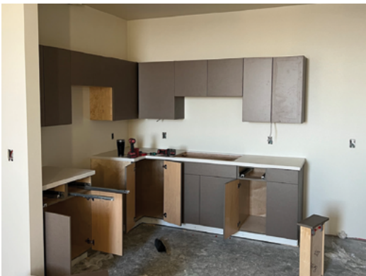
Casework mock-up (Feb 2025)
