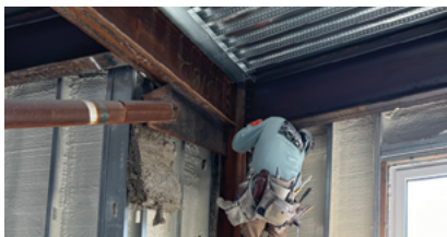
Installation of rock wool at exterior
