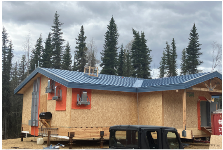
Anvik Clinic roofing and siding
