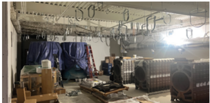
Mechanical room equipment rough-in
