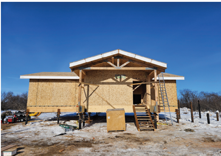
Oscarville Clinic exterior construction
