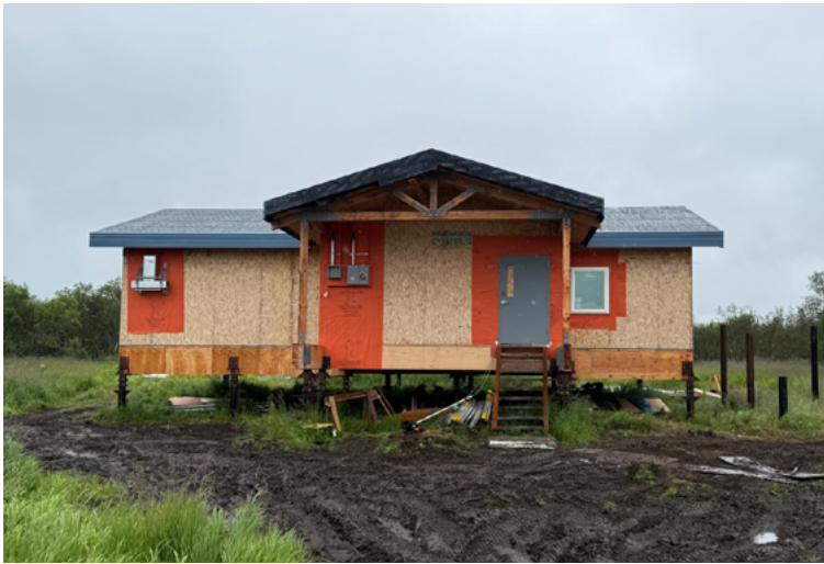
Oscarville Village Clinic construction
