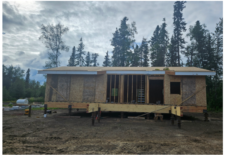
Stony River Village Clinic construction
