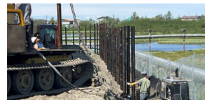
YKHC driving pile for retaining wall
