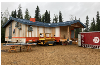
Anvik Village Clinic construction
