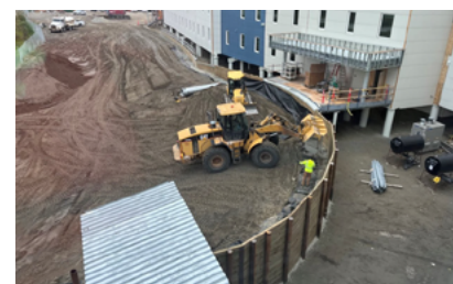
Backfill retaining wall at main entry
