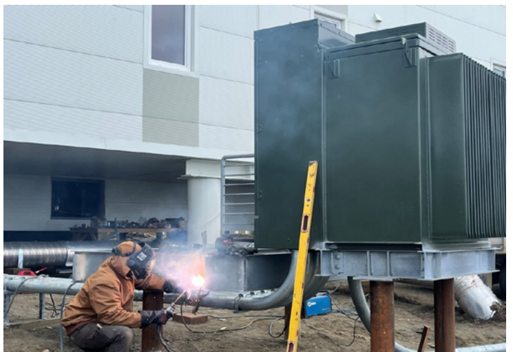
Tuntu Apartments - Fabricating steel platform for transformer access
