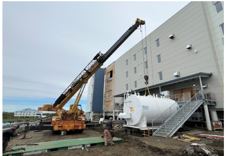
Tuntu Apartments - Setting above ground fuel oil storage tank
