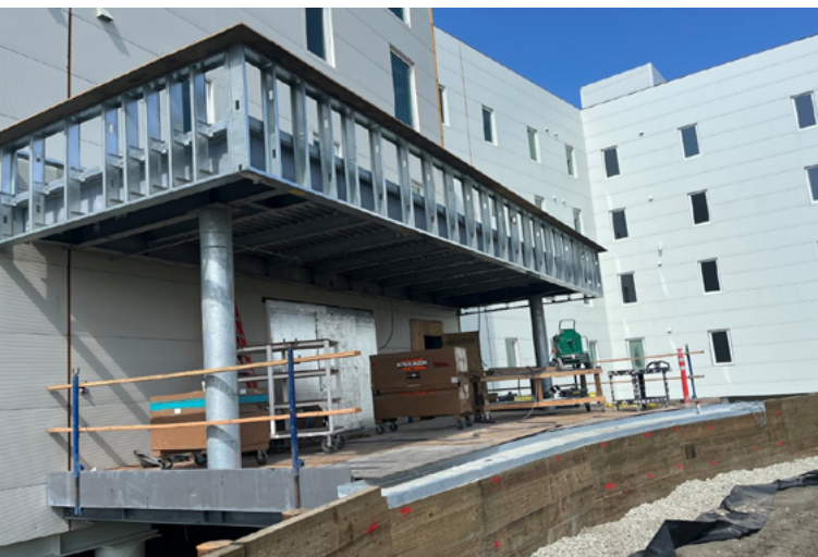
Tuntu Apartments - Main entry canopy framing
