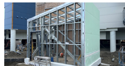
Framing the lift station enclosure
