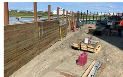
Installing treated wood walers on piling
