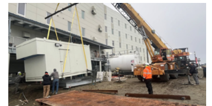
Setting building standby generator
