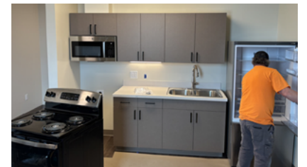
YKHC installing refrigerators and ranges
