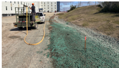
Topsoil and hydroseed
