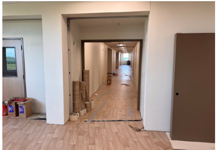
Tuntu Apartments: Lobby and corridor flooring.
