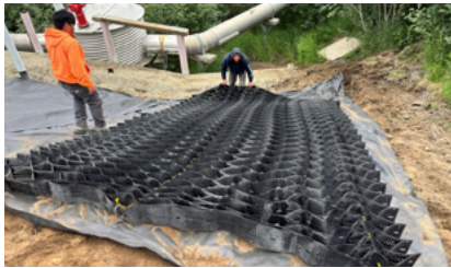
Geoweb slope stabilization
