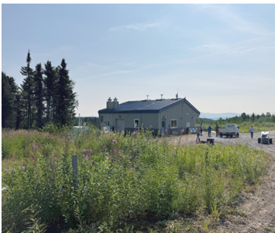
At the request of the tribe, the new clinic room in Lime Village was added as part of the existing washeteria building. YKHC works closely with tribes to ensure each clinic meets the needs of the community.
