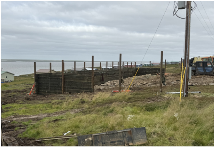
Mertarvik Health Clinic - Civil and foundation work started.
