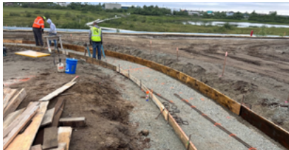
Formwork for west parking lot sidewalk
